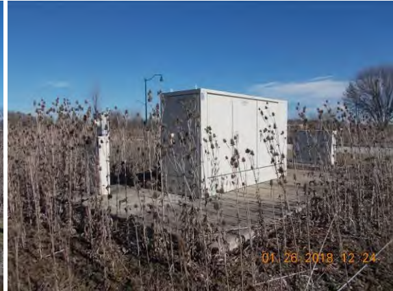
Pad-mounted transformers at northwest property line
