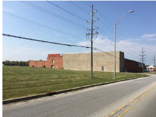
Subject Property North and East Elevations
