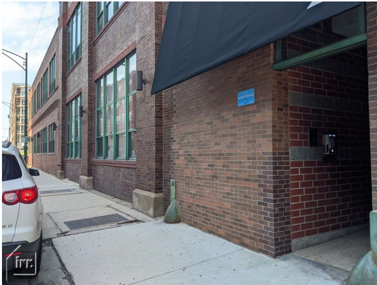
Commercial Condo Unit - Unit 105 22 N. Morgan St, Unit 105 Chicago, Illinois
