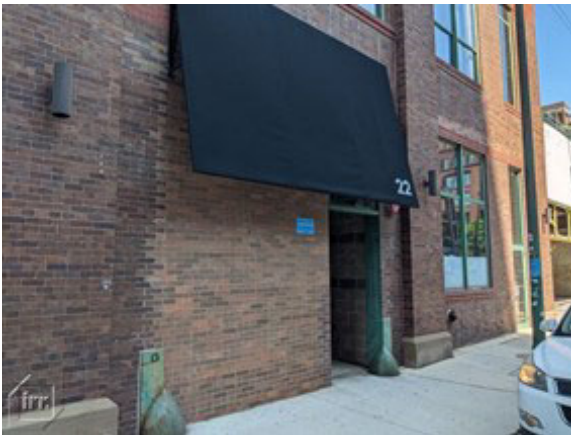
Entry to Building - Subject door to be installed at left
