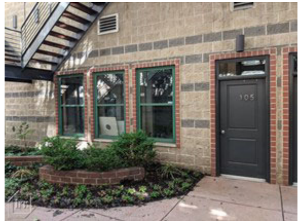
Subject courtyard entry door
