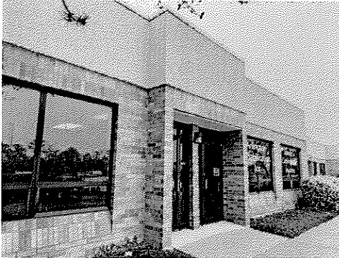
Front facade entrance
