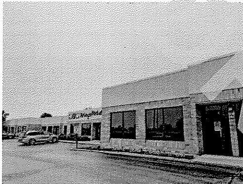
West facing facade
