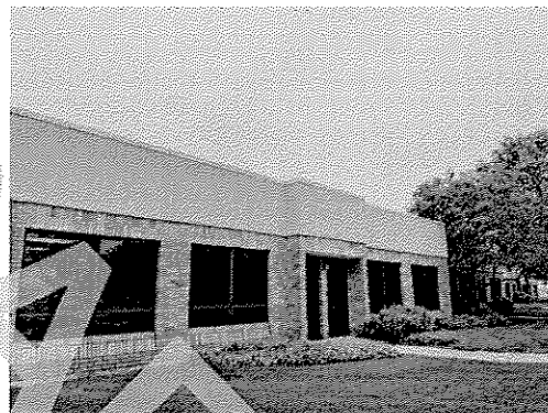
East facing facade
