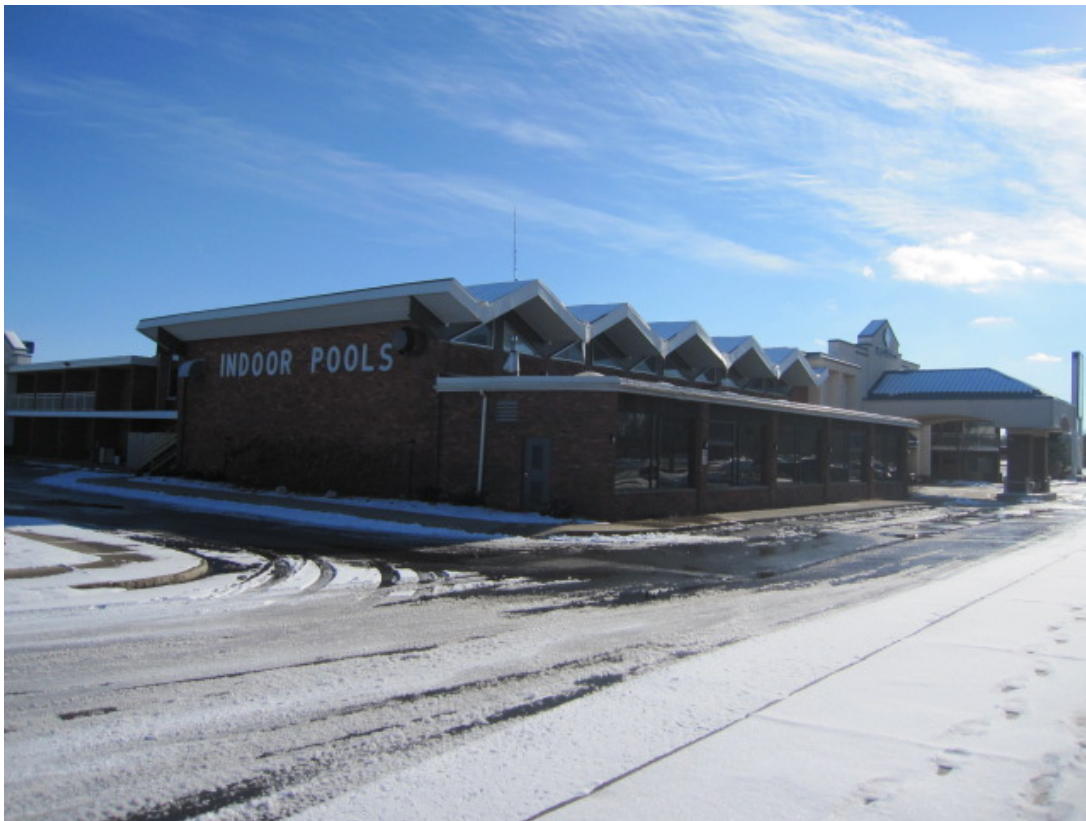
View of the Building from Northwest
