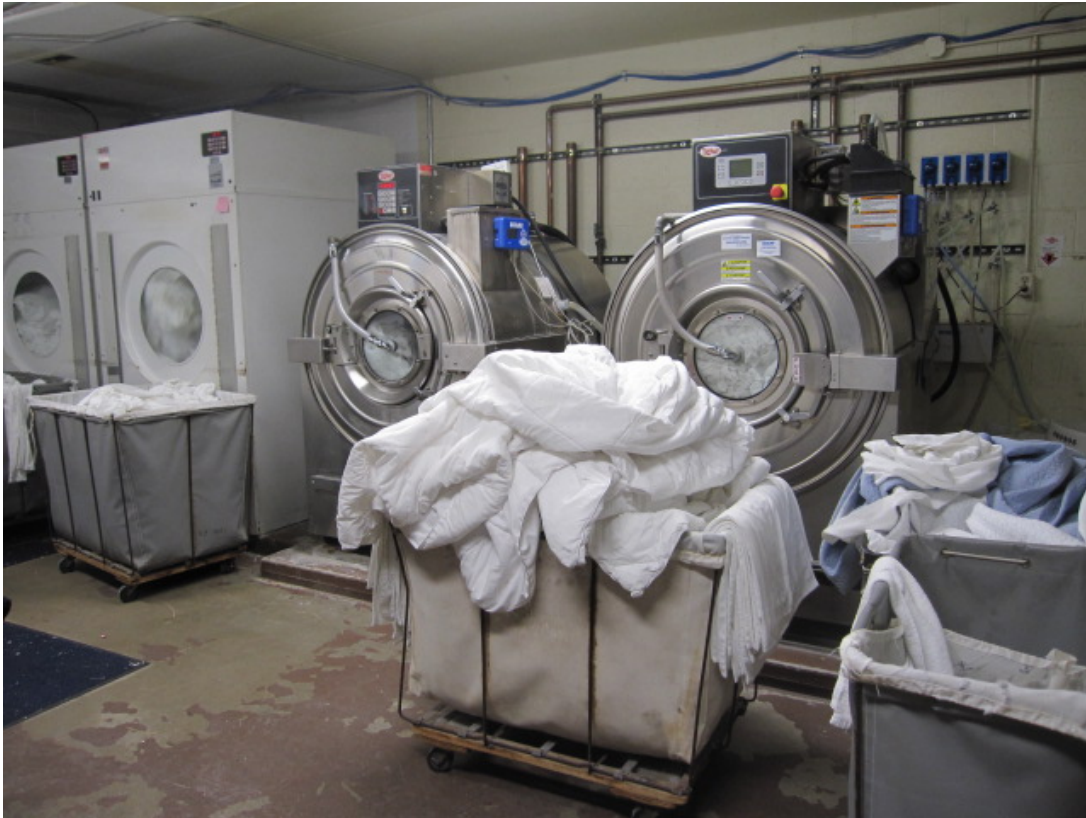
View of the Laundry Room
