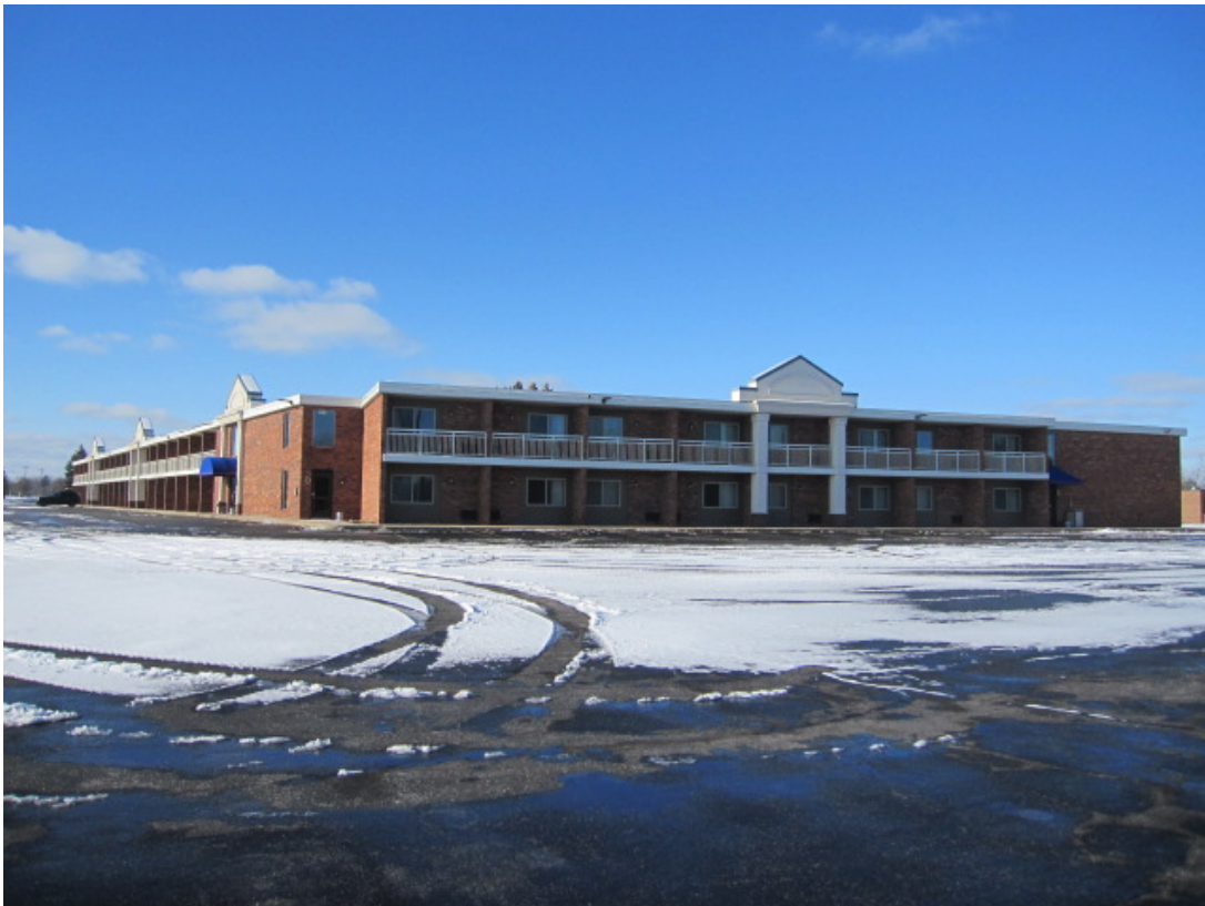
View of the Building from Northeast
